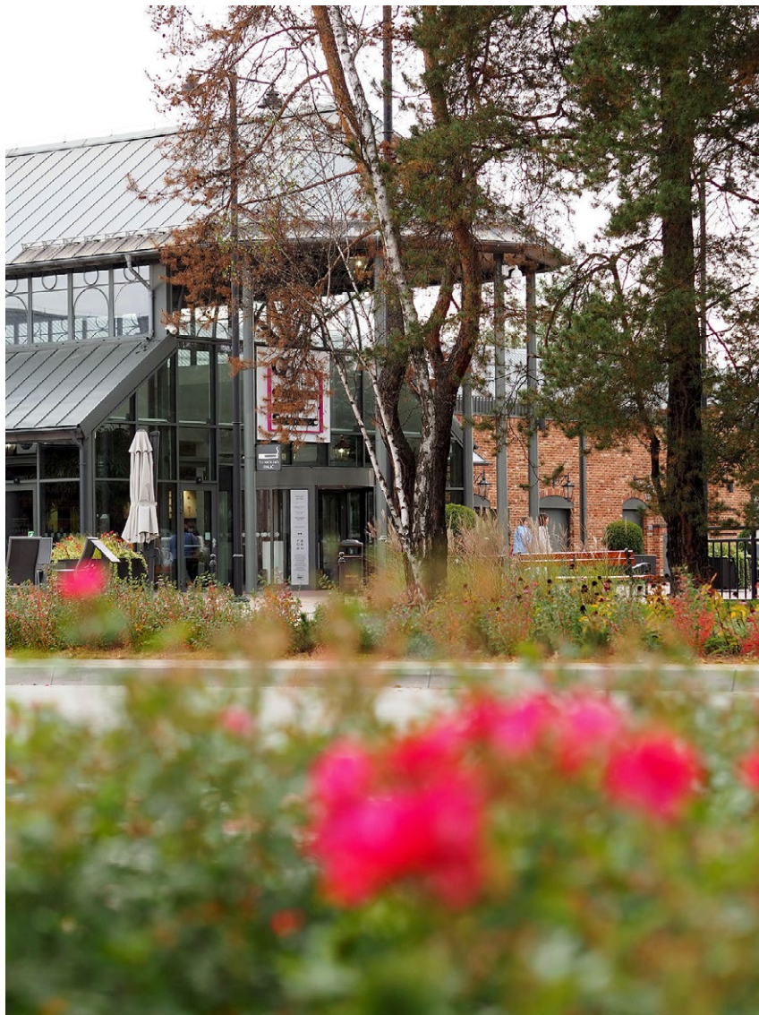
Designer Outlet Sosnowiec | Fot. ROS Retail Outlet Shopping
